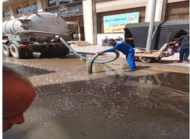
Fig. 5. Sewage overflow in a number of locations in the city center of Karbala
